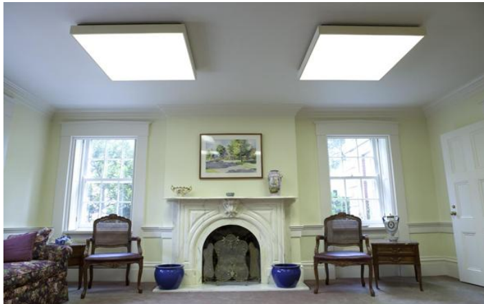
Borealis T8 LED Tube Lighting Installation
